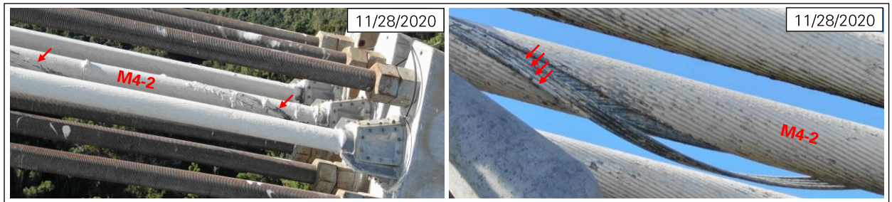
Figure 28: M4 cables near platform on November 28, 2020, with no visible change since November 7, 2020 (photos: NAIC Arecibo Observatory, a facility of the NSF).
