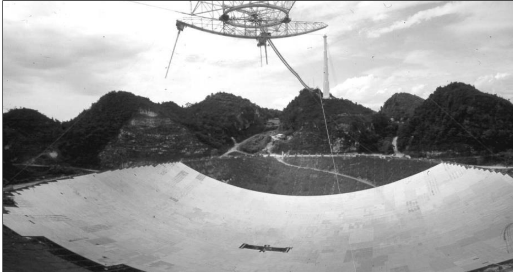
Figure 8: Aluminum panels being installed on the primary reflector during the first upgrade (photo: NAIC Arecibo Observatory, a facility of the NSF).
