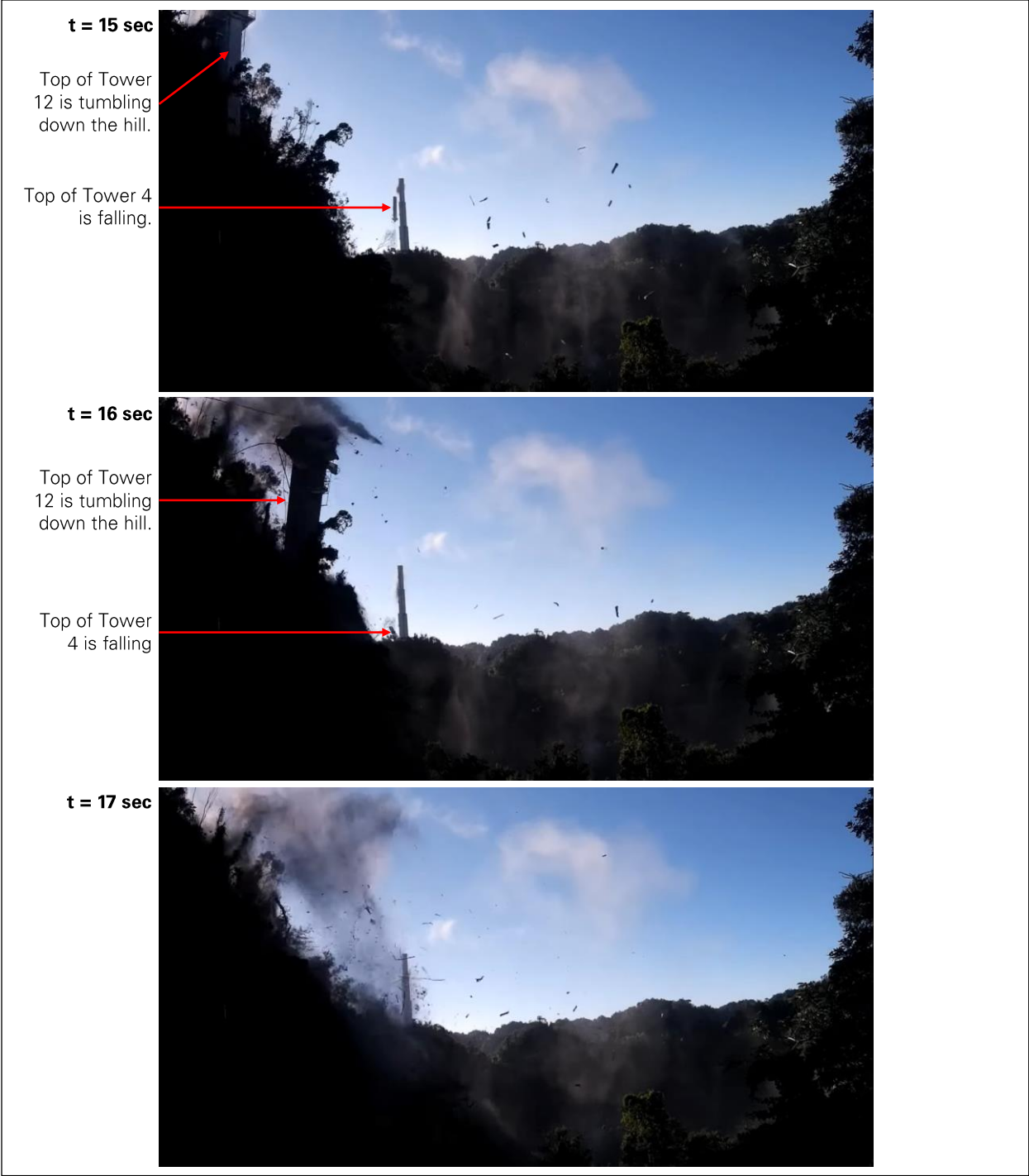
Figure 39: Still images of telescope collapse video: seconds 15 to 17 (video: NAIC Arecibo Observatory, a facility of the NSF).
