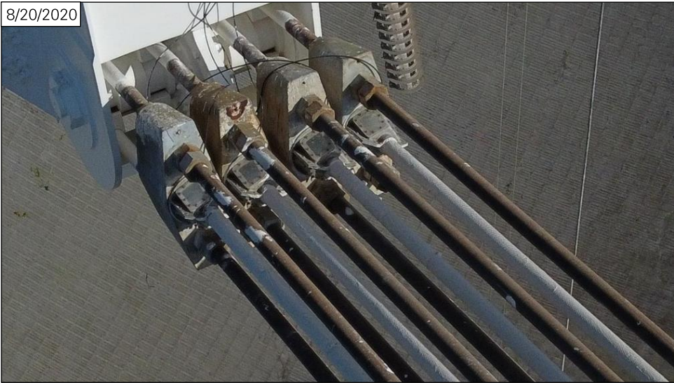
Figure 5: M4 cable near platform on August 20, 2020. No wire is broken. (Photo: NAIC Arecibo Observatory, a facility of the NSF.)
