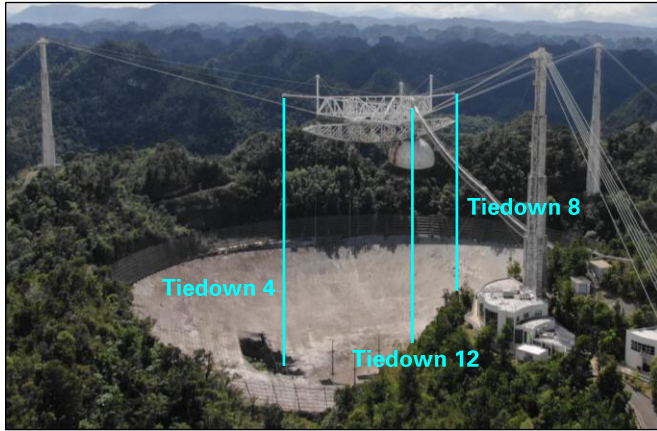
Figure 6: Upgraded structure tiedowns (photo: NSF).
