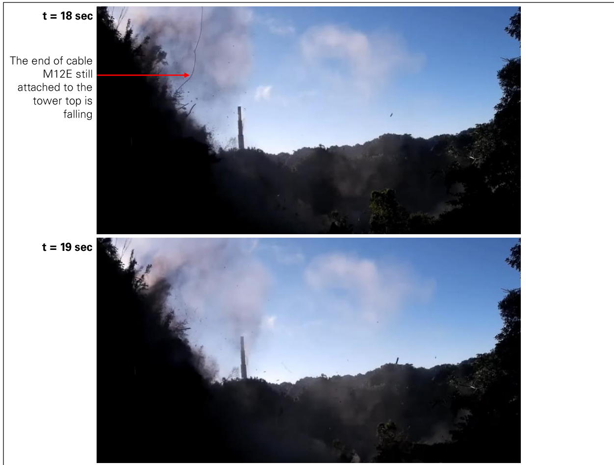
Figure 40: Still images of telescope collapse video: seconds 18 to 19 (video: NAIC Arecibo Observatory, a facility of the NSF).
