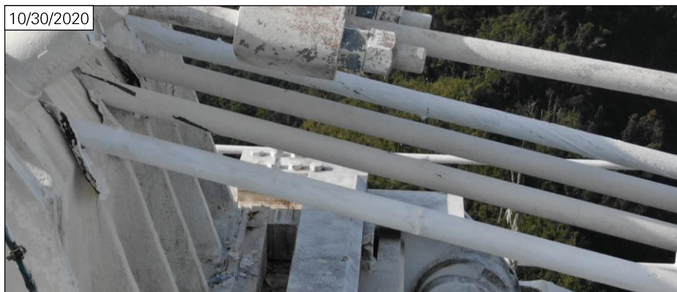
Figure 12: M4 cables near Tower 4 on October 30, 2020. No significant change is visible since October 19, 2020. (Photo: NAIC Arecibo Observatory, a facility of the NSF.)
