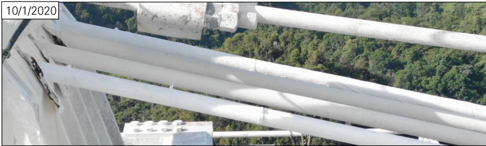
Figure 9: M4 cables freshly repainted near Tower 4 on October 1, 2020 (photo: NAIC Arecibo Observatory, a facility of the NSF.)
