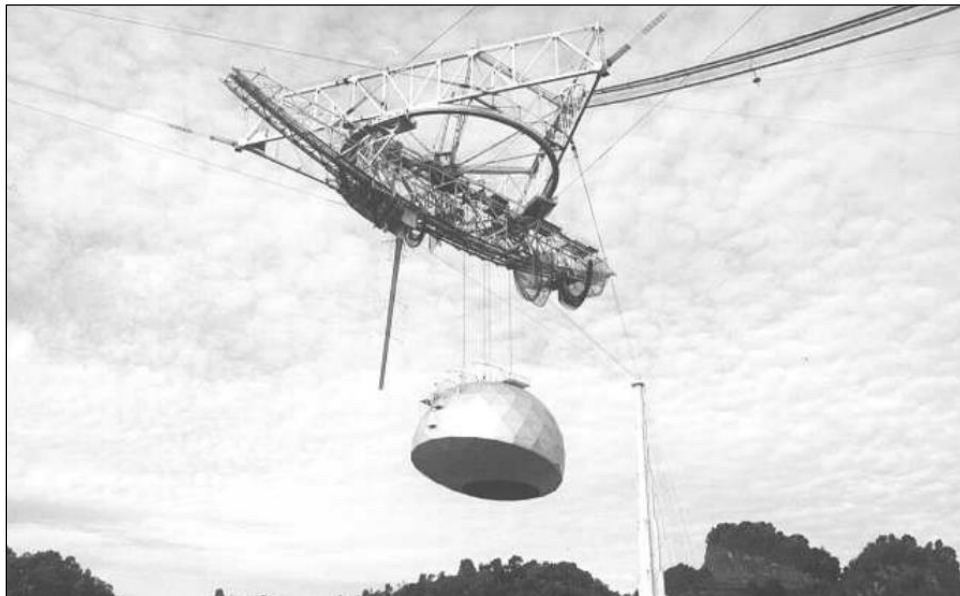
Figure 13: Gregorian being lifted into place during second upgrade (photo: NAIC Arecibo Observatory, a facility of the NSF).
