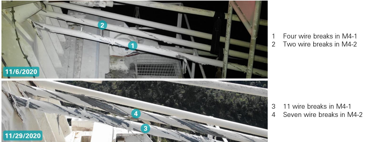
Figure 27: Wire break development after second cable failure (photos: NAIC Arecibo Observatory, a facility of the NSF).
