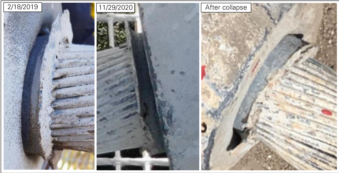
Figure 21: Cable slip at socket M8N_T (left and center photos: NAIC Arecibo Observatory, a facility of the NSF).
