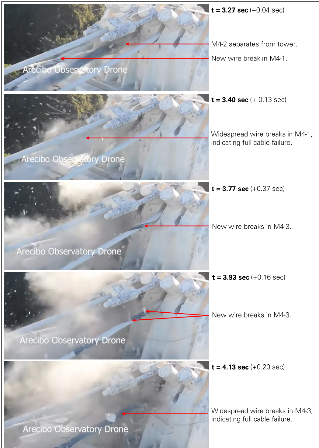
Figure 32: Still images of drone video of top of Tower 4 during telescope collapse: seconds 3.27 to 4.13 (video: NAIC Arcibo Observatory, a facility of the NSF).
