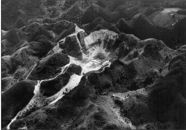
Figure 1: Telescope site during partial excavation of hills around the natural sinkhole in December 1960 (photo: NAIC Arecibo Observatory, a facility of the NSF).
