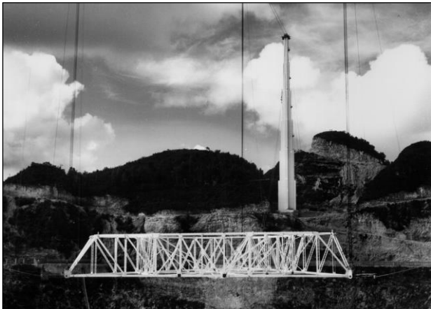
Figure 4: Platform being lifted into place in October 1962 (photo: NAIC Arecibo Observatory, a facility of the NSF).
