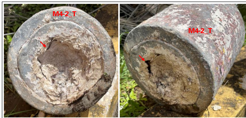
Figure 34: Socket M4-2_T recovered after collapse.
