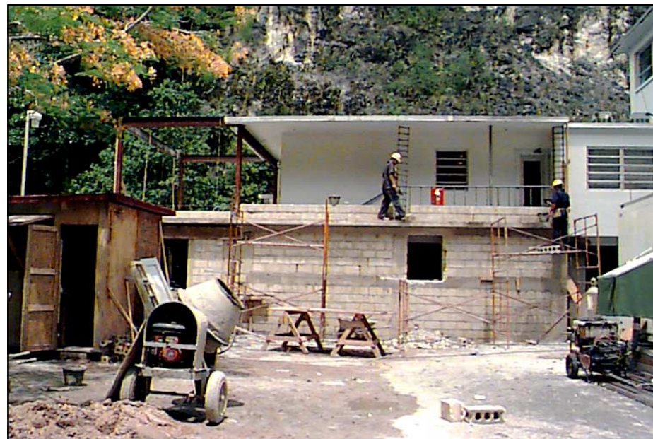
Another angle on the Control Room construction.
