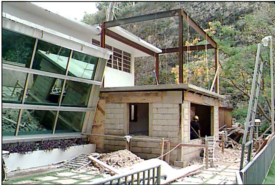
Construction on the Control Room extension.
