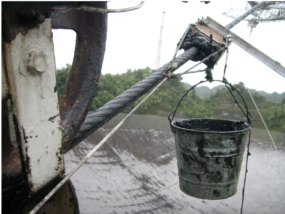
Photo 4 – Removing excess grease from track rope with groove cleaner.
