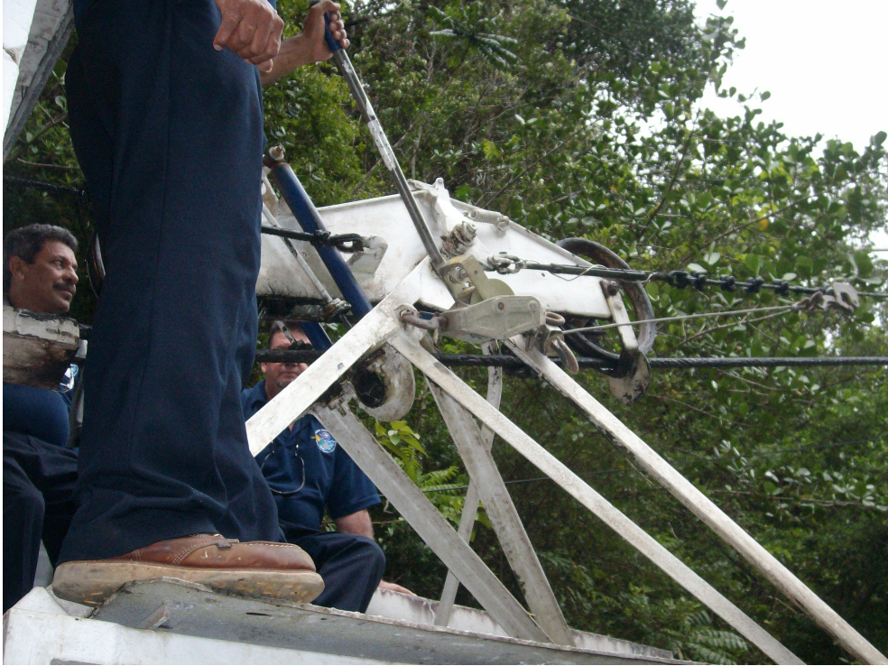
Photo 3 – Performing slack rope test of track cable brake.
